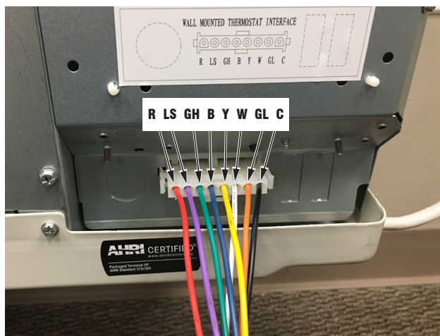
Figure 44 Remote Thermostat Harness Connected
